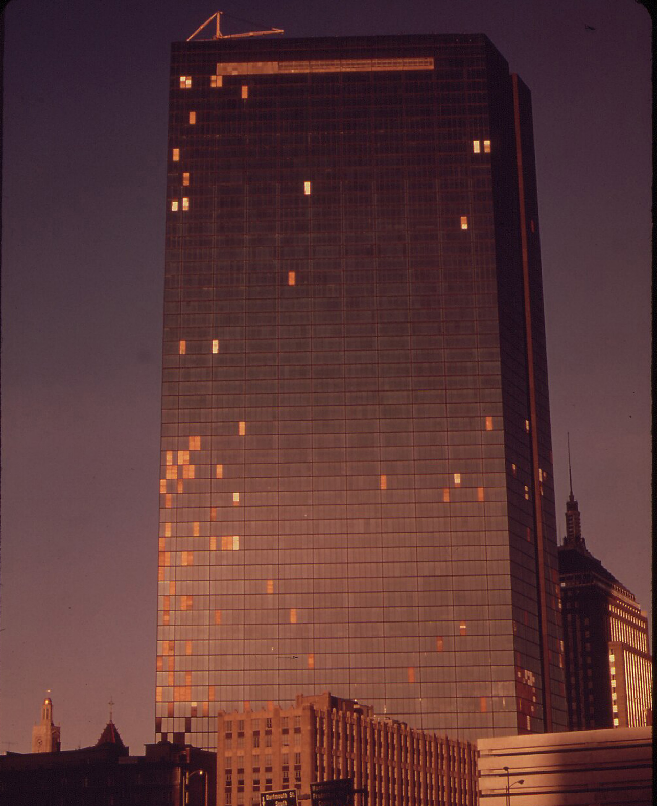
Figure 28. The John Hancock Tower with broken windows, 1973. (US National Archives)
