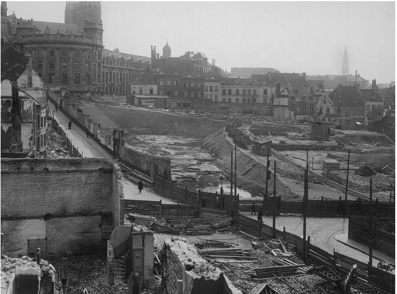
Figure 1. In 1912, public works were underway, particularly for the construction of the North-South railway junction. This required the erasure of entire city blocks, leading to a multitude of simultaneous demolitions (KIK-IRPA, Brussels).
