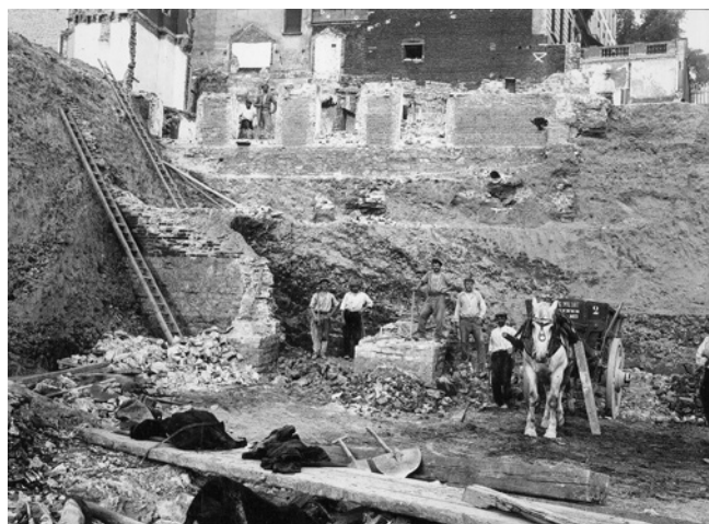
Figure 6. Demolishers using tools like ladders, shovels, pick axes, and wheel carts during demolition works in 1911 (KIK-IRPA, Brussels).
